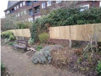
Fencing renewal ( Ingram Crescent )
